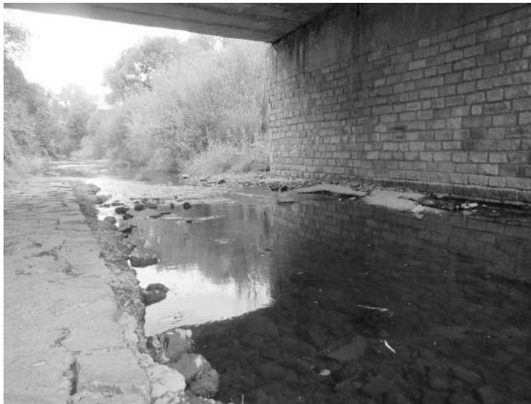
Fig. 6-3. Corridor for otter movement under bridge in Czech. It reduce otter casualties by vehicle.
